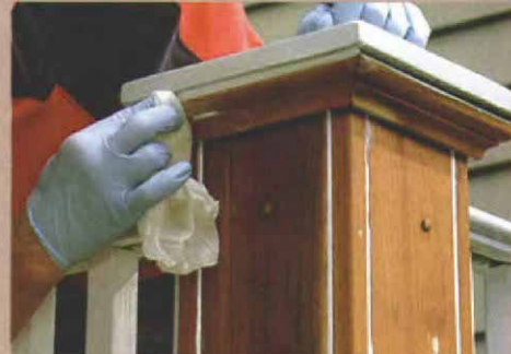
2. Mineral spirits remove excess caulk.
