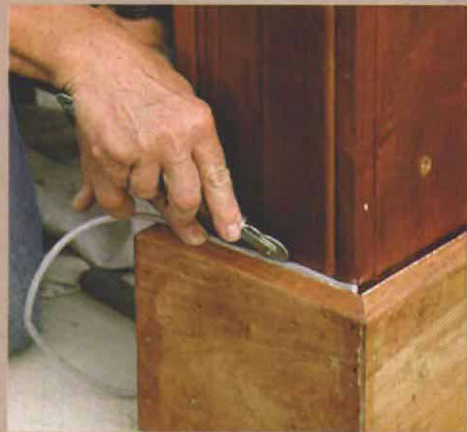
3. Backer rod allows caulk to flex.
