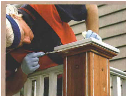
1. Palette knife tools visible joints.
