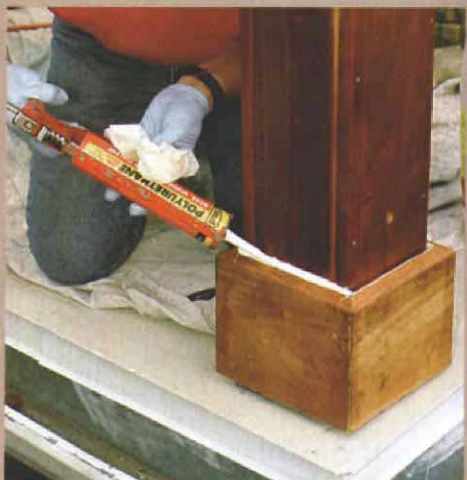
4. Polyurethane is the first line of defense.
